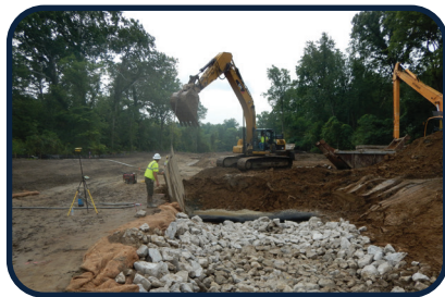
Construction of fishway begins.
