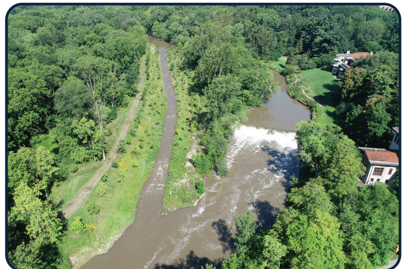
Aerial of HFE Dam and fishway after restoration
