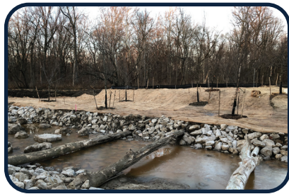
Logs are placed to create habitat in the riffles and pools.
