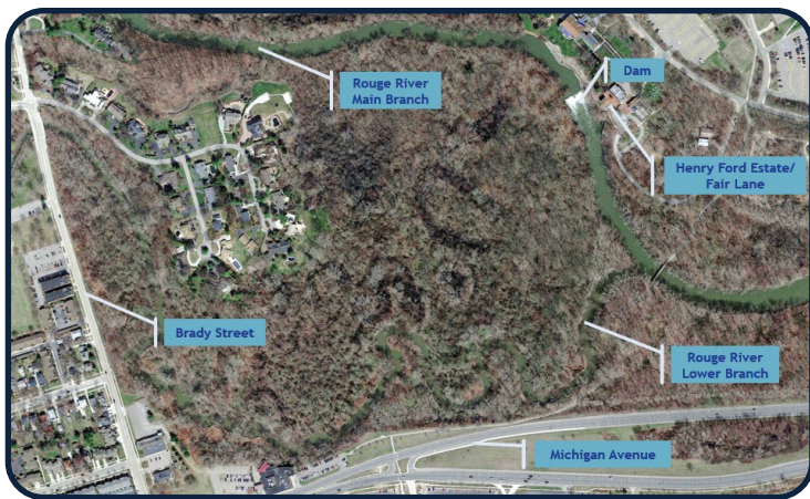
Aerial of HFE Dam before restoration
